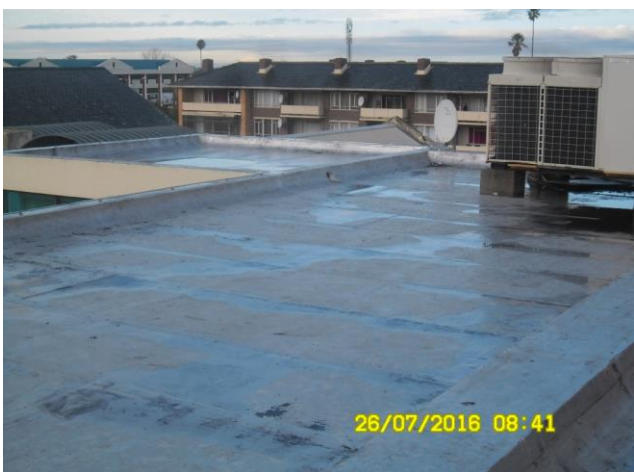
Application of 4mm bitumen membrane torch-on waterproofing system
